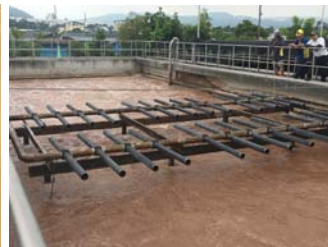
Pulp/paper, 20000m 3 & 30000m 3 aeration tank
