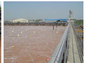
Pulp/paper, 20000m 3 & 30000m 3 aeration tank
