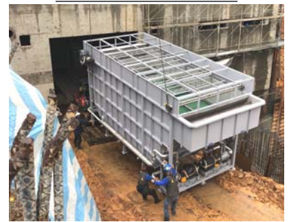
250m 3 /hr (TT River clarification)
