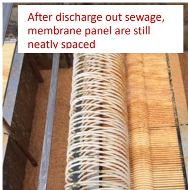
↑ High toughness and clog preventing membrane tube diffuser in aeration case.
